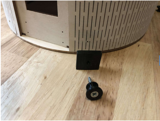
The plate goes on the inside, and is meant to divide the force over a larger area
